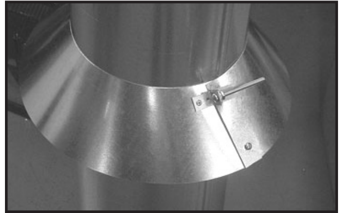
Figure 7.12 Insert Bolt into Brackets
