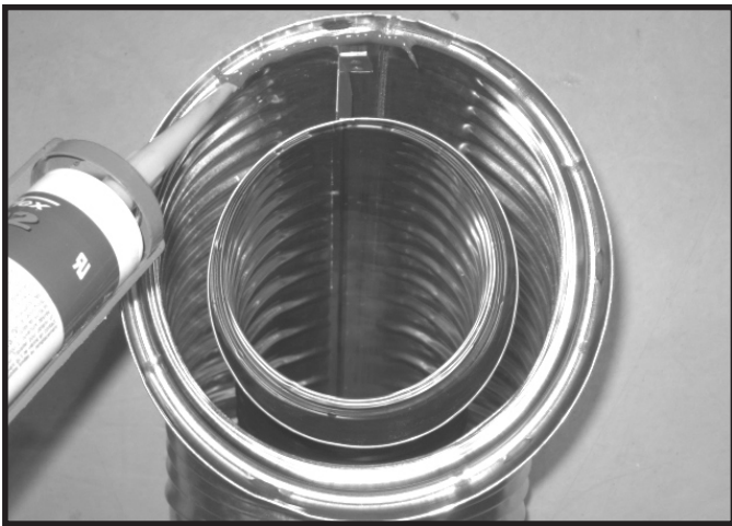
Figure 7.1 High Temperature Silicone Sealant
